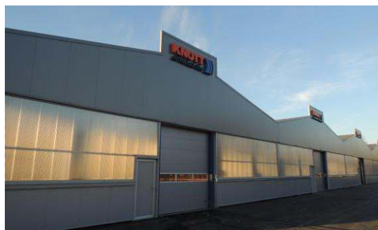
Knot Autoflex, Bečej - polikarbonatne fasade
